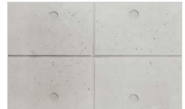
LightBeton® Formwork System transfers detailed impressions into the surface of the concrete
